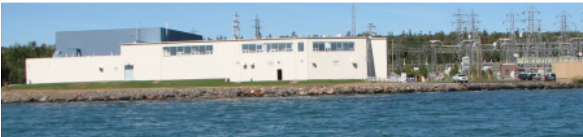
Bare Point Water Treatment Plant
