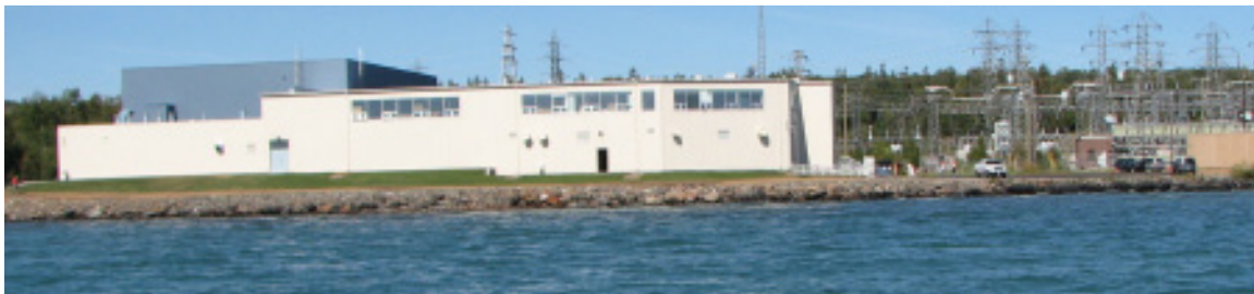
Bare Point Water Treatment Plant
